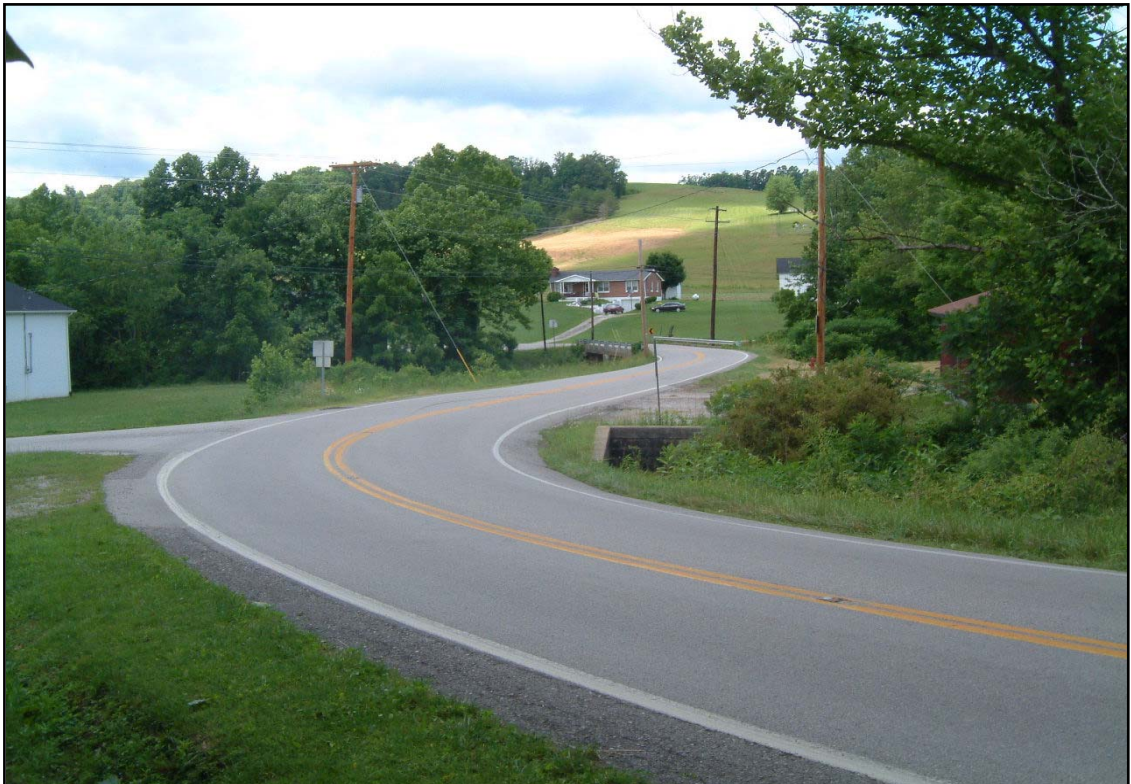
Photo 8. Bridge on KY 30 near Traveller's Rest
