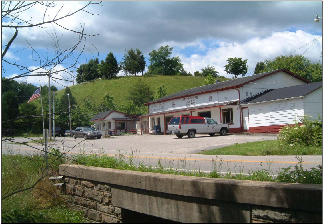
Photo 5. KY 30 at Vincent (Brushy Creek) (looking south)
