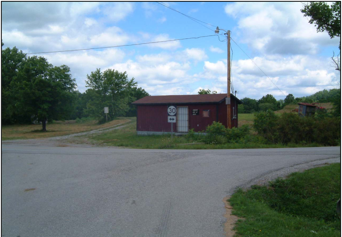
Photo 6. Structure along KY 30 near Traveller's Rest
