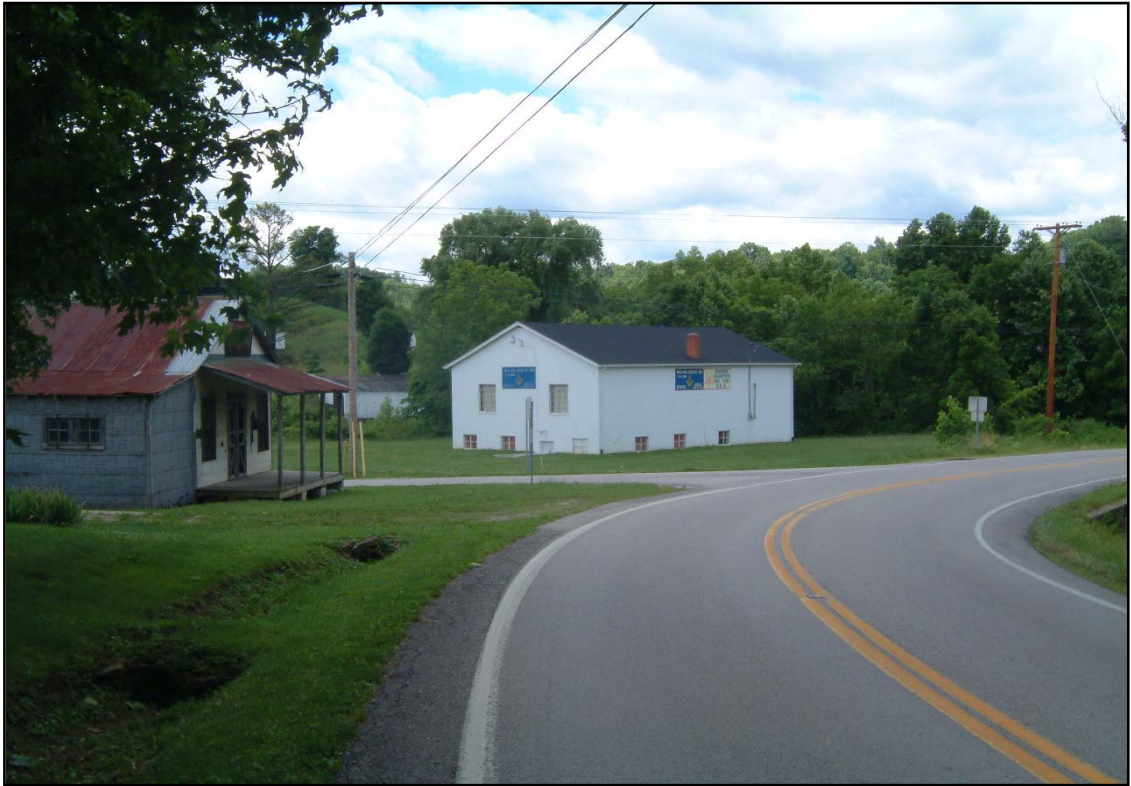
Photo 7. Residences along KY 30 near Traveller's Rest
