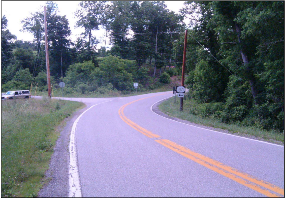
Photo 11. KY 30 at KY 1071, near Green Hall (looking north)
